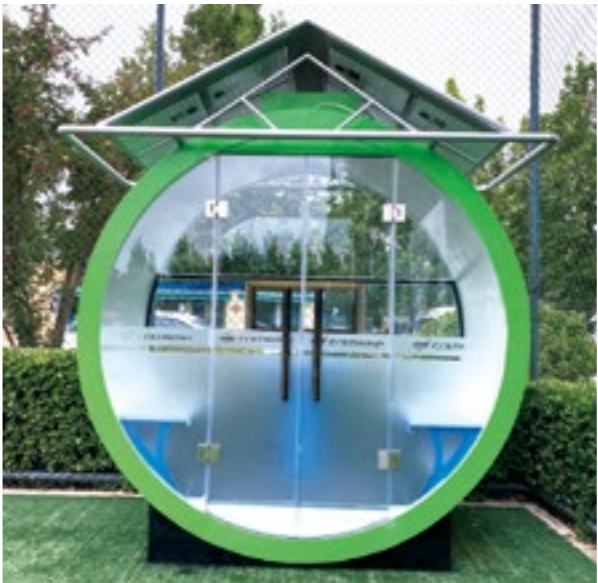
The meeting rooms have been made of the root of decommissioned blades. Photovoltaic panels and energy storage devices have been installed on roofs to provide power for lighting in the rooms.
