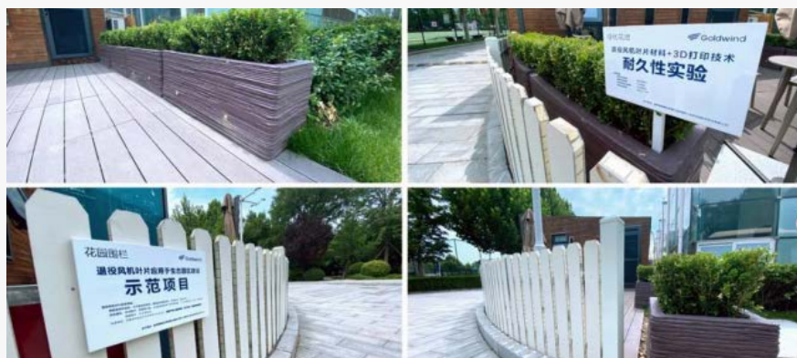
Waste blades were transformed into the raw materials for 3D printing to build a flower bed
