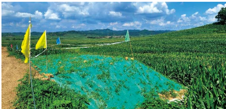
Topsoil is stripped, collected, stacked and covered centrally
